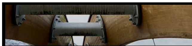
Reusssteg Pedestrian Bridge over the Reuss River, Seedorf-Flüelen, Canton Uri, Switzerland
