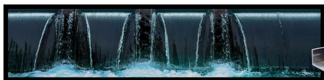
Spreuerbrücke Bridge Dam on the Reuss River Lucerne, Switzerland
